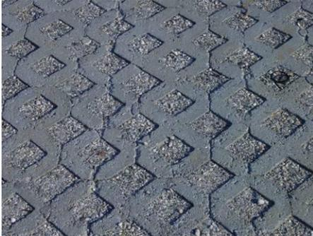
Pervious paving infiltrates stormwater back into the soil thereby recharging groundwater.
