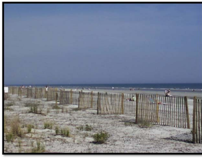
FIGURE 30: SAND FENCING
