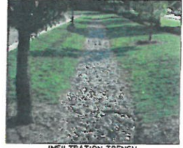
INFILTRATION TRENCH
