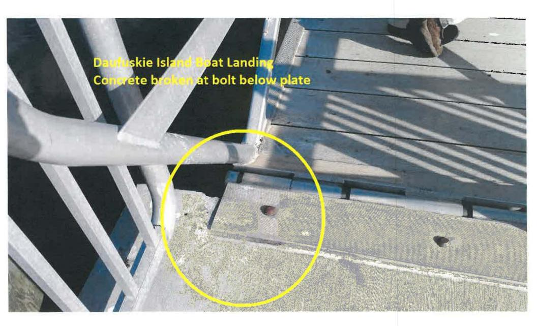
Daufuskie Island Boat Landing Broken float deck & structure
