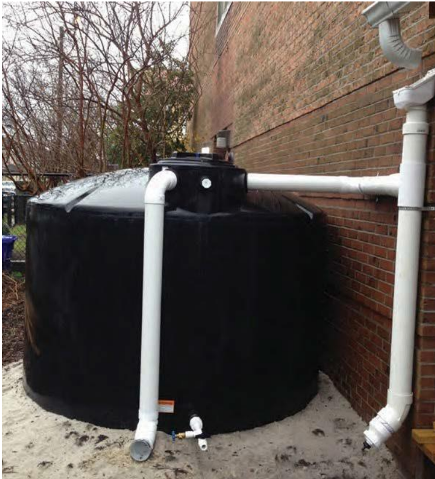
Figure 4.23. Example cistern application (photo: Marty Morganello).
