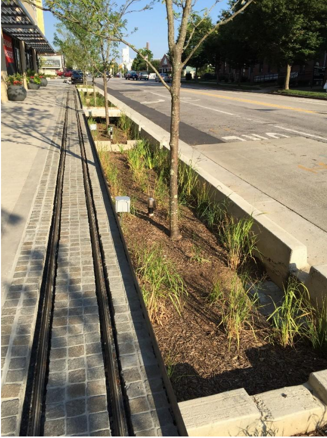
Figure 4.5. Example streetscape bioretention.
