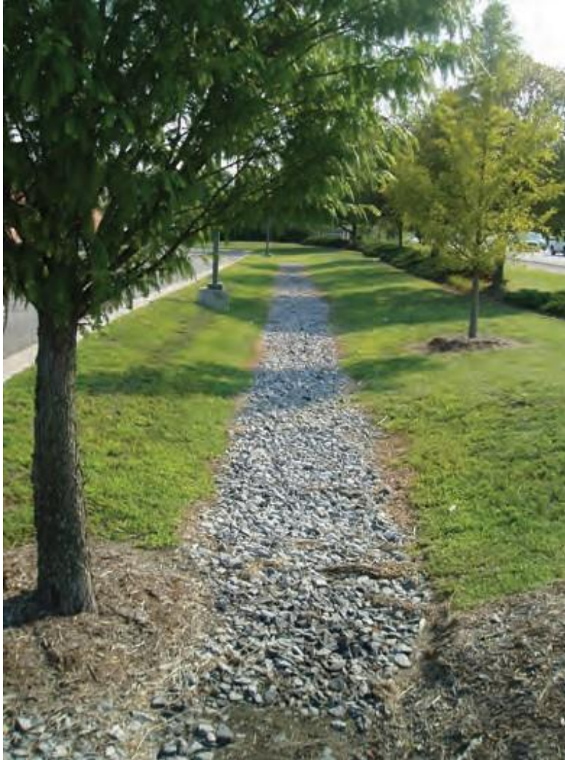
Figure 4.16. Infiltration practice in median strip.
