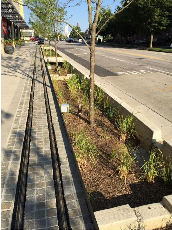
Figure 4.5. Example streetscape bioretention.
