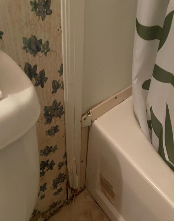
Water damage on the opposite of toilet on floor and wall panel
